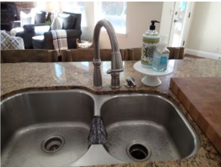
Suggest caulking as necessary.
