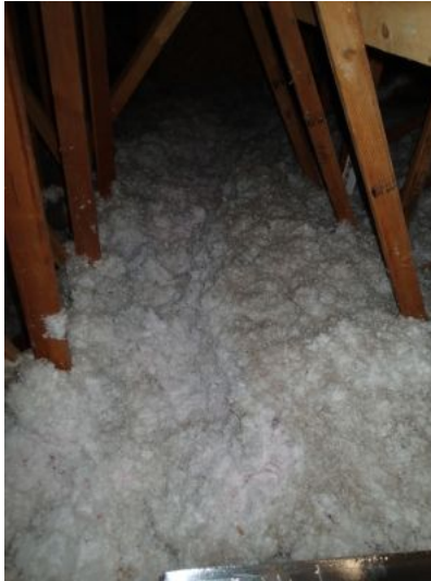
Insulation appears adequate.
