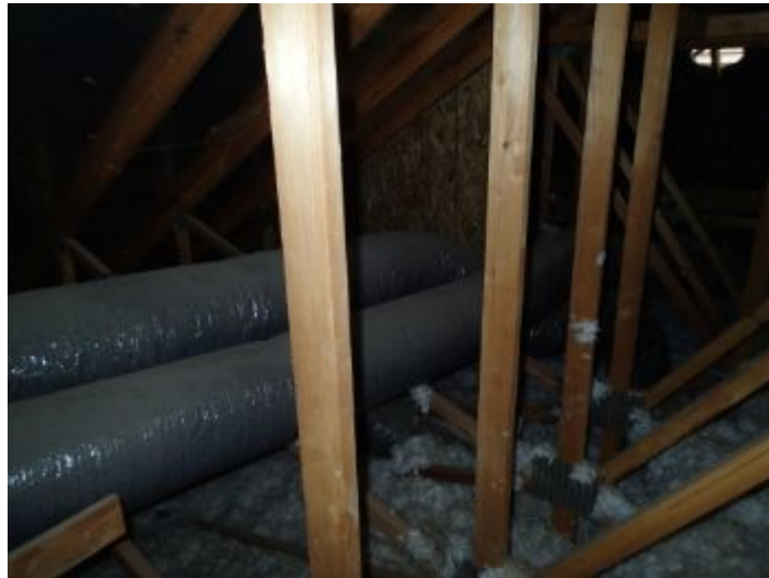
Ducts appear to be in good shape at the time of inspection.
