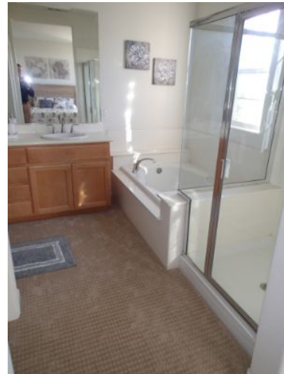
Carpet is not recommended in bathrooms due to potential to harbor moisture, which could lead to unwanted mold issues. Master bath.
