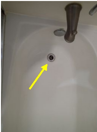
Stopper is missing.
