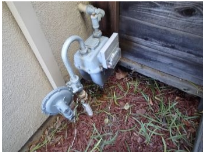
Located on the north side near the garage.
