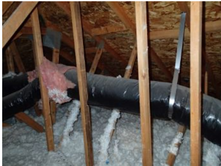
Visible structural components appeared to be functional at time of inspection.
