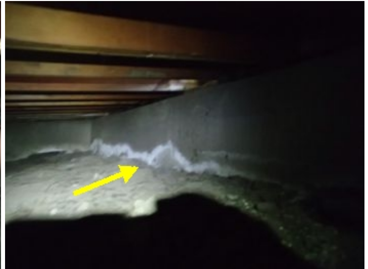
Efflorescence observed; this is a mineral deposit left behind from previous exterior water infiltration.
