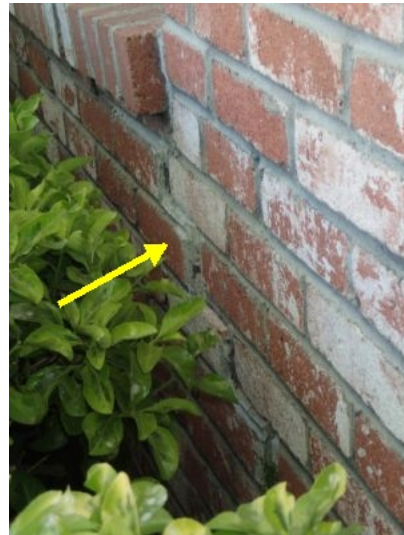
Caulk and seal all gaps, cracks and openings.
