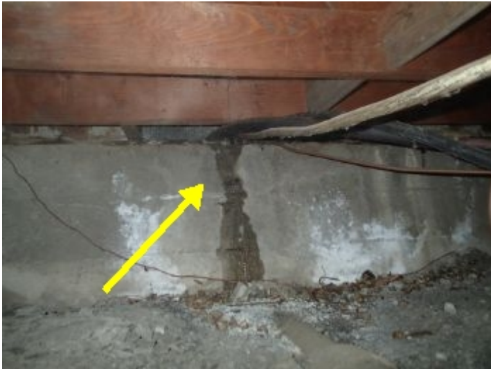
Active leaks observed at the time of inspection. It appears to be from the A/C condensation line.
